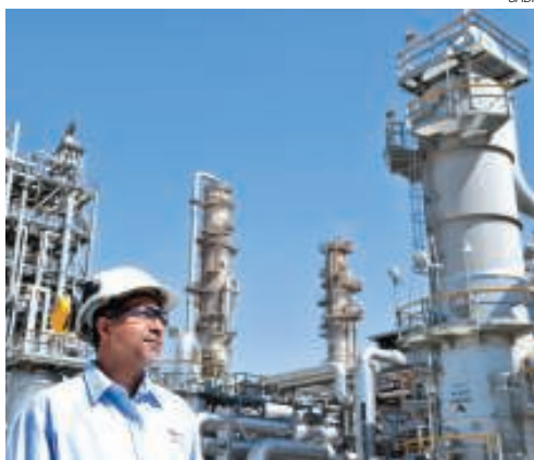
FIGURE 1. SABIC's United CO 2 purification plant captures carbon dioxide from an ethylene glycol process and distributes it as a raw material to other production units
